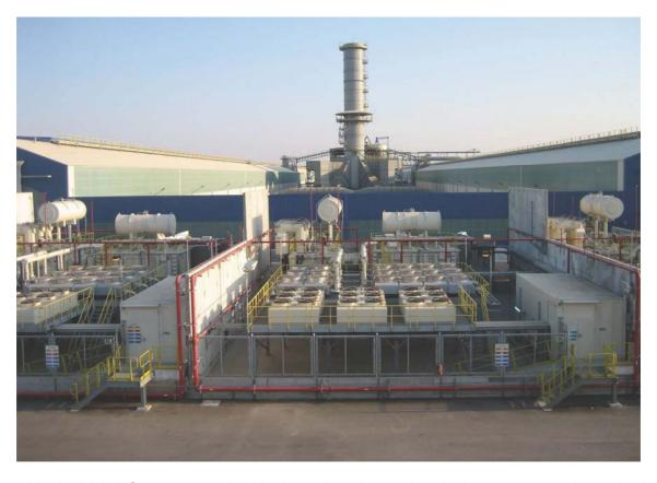
To provide the high DC current required by intensive electro-chemical processes such as aluminium smelting, multiple high-power rectifiers are typically connected in parallel so that together, they can provide very high current.
